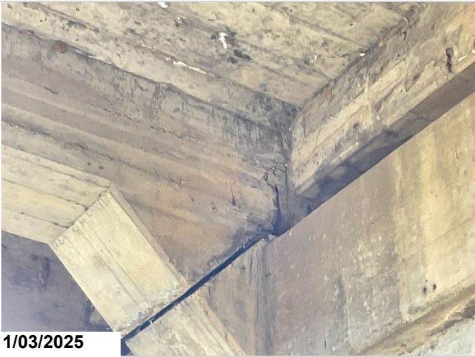
Span # 6, Bent # 6, Girder # 4: Shallow 5" high spall with exposed reinforcing steel. Exposed steel 1LF CS3.
