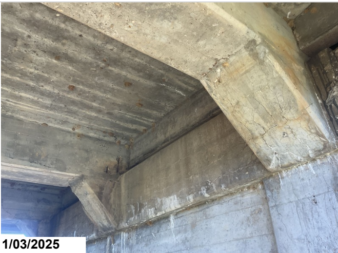
Span # 1, Girders # 3 and 4, At Bent # 2: Mapcracking in haunch, girder # 3 has spalls with exposed steel. Cracking 1LF CS3, Exposed steel 1LF CS3.
