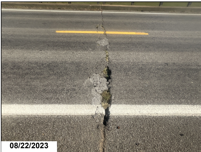
Asphalt over bent # 5 coming apart with potholes forming in the driving surface.
