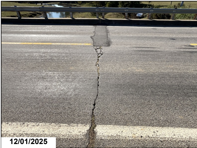
Bent # 2 Expansion Joint: Asphalt breaking apart.
