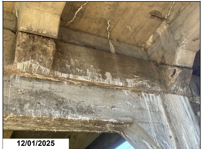
Bent # 2, Cap, Ahead Side: Haunches under Girders # 2 and 3: Map cracking with spalling and exposed steel.
