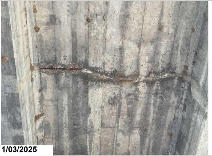
Span # 7, Bay # 2: Transverse cracking with efflorescence and spalling with exposed reinforcing steel. Efflorescence 5SF CS2, Exposed steel 2SF CS3.
