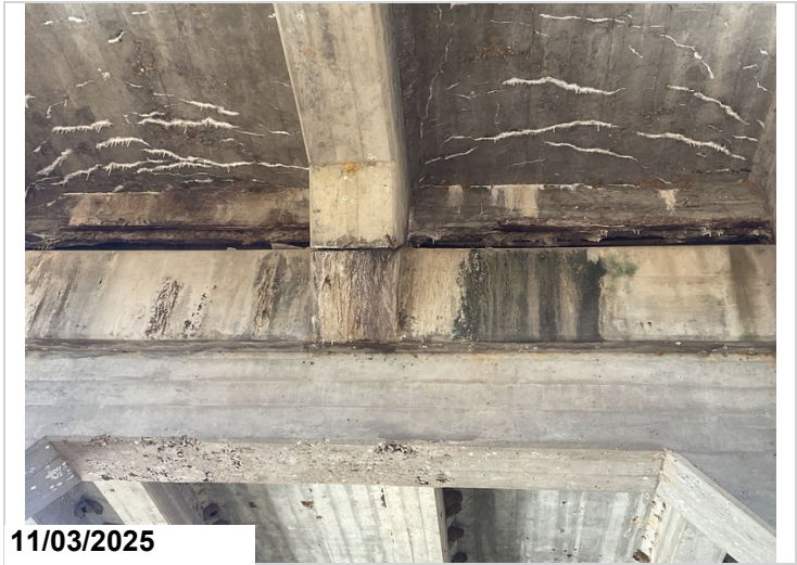
Span # 4, Over Bent # 4: Spalling with exposed reinforcing steel in expansion dam. Exposed steel 10SF CS3.
