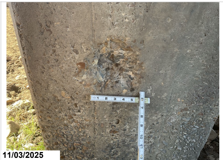
Bent # 6, Column # 2, Ahead Side: 6" spall with no exposed reinforcing steel. Spall/ delam 1EA CS3.
