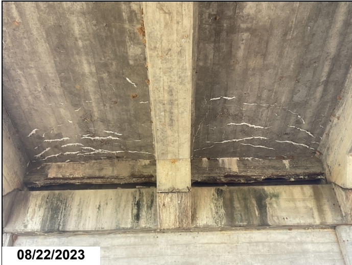
Span # 4 over bent # 4-Spalling with exposed reinforcing steel in expansion dam.
