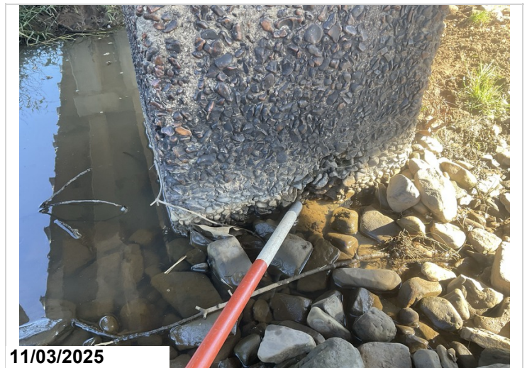
Bent # 5, Column # 2: Concrete deterioration/ heavy abrasion. Abrasion 1EA CS3.
