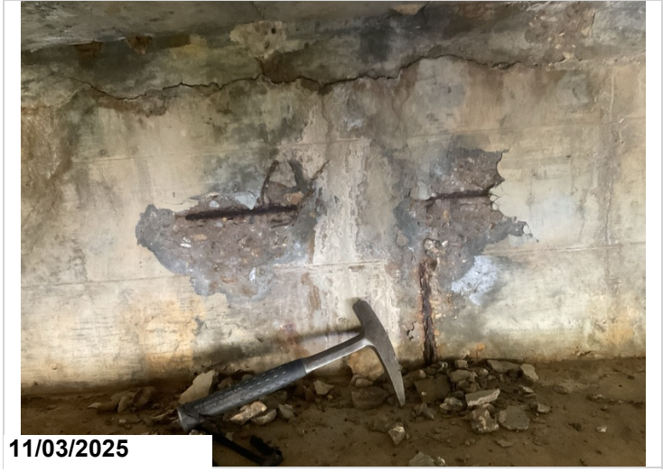
Span # 1, At Abutment # 1: Girder haunches have horizontal cracking with delaminated areas.
