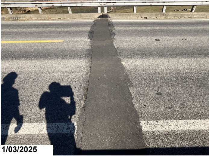
Bent # 6 Expansion Joint: Asphalt patch over joint.
