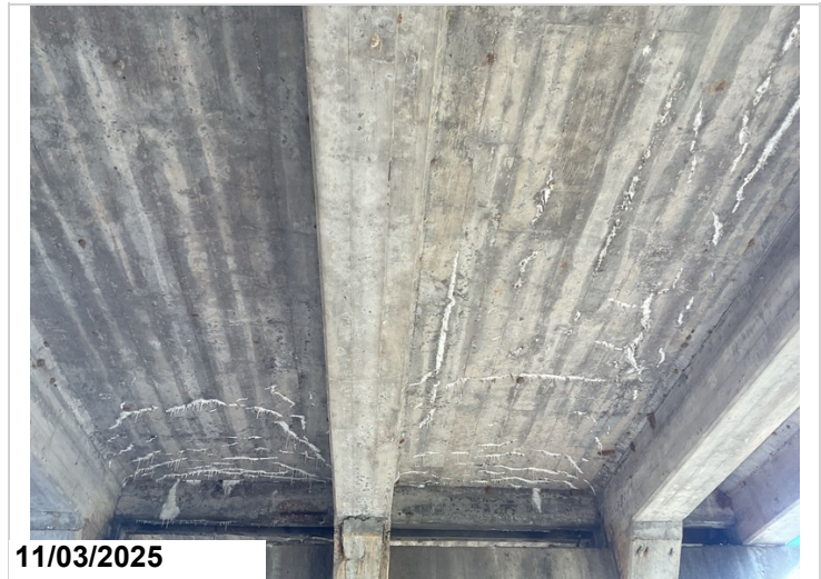
Span # 7, Bays # 2 and 3: Cracking with efflorescence.
