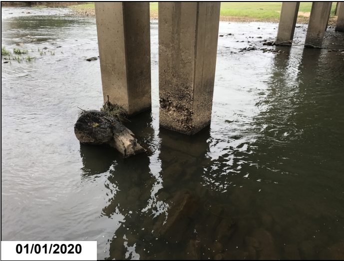
Bent # 3, column # 2 has concrete deterioration with exposed reinforcing steel.
