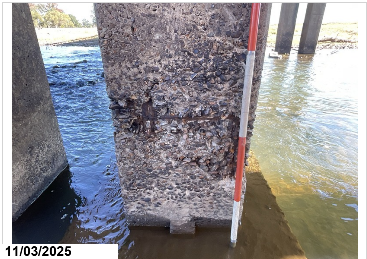
Bent # 3, Column # 2, Back Side: Full width x 15" high area of concrete deterioration with exposed reinforcing steel and up to 2" of concrete section loss. Exposed steel has section loss. Exposed steel 1EA CS3
