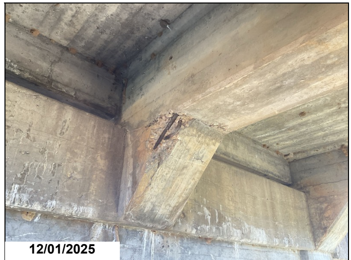
Span # 1, Girders # 3 and 4, At Bent # 2: Map cracking in haunch, girder # 3 has spalls with exposed steel.
