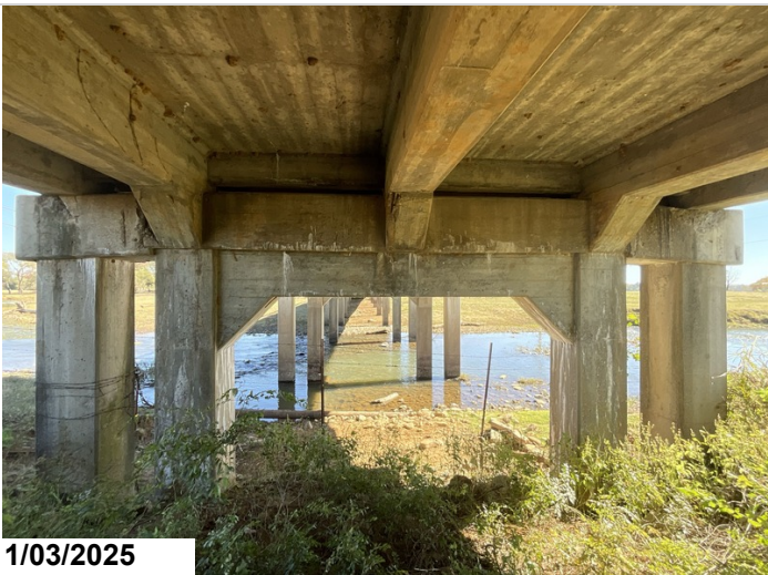
Bent # 2 Cap, Back Side: Mapcracking with efflorescence and spalling with exposed steel.
