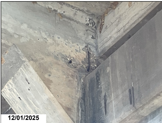
Span # 5, Bent # 6, Girder # 3: Shallow spalls with exposed reinforcing steel.
