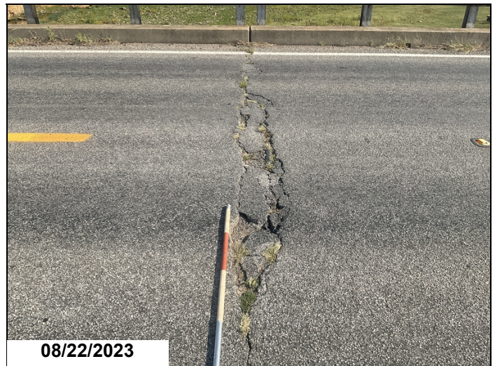
Asphalt over bent # 4 coming apart with potholes forming in the driving surface.
