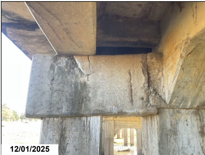
Bent # 2 Cap, Left Back Side: Spall/ delaminated areas and exposed steel.
