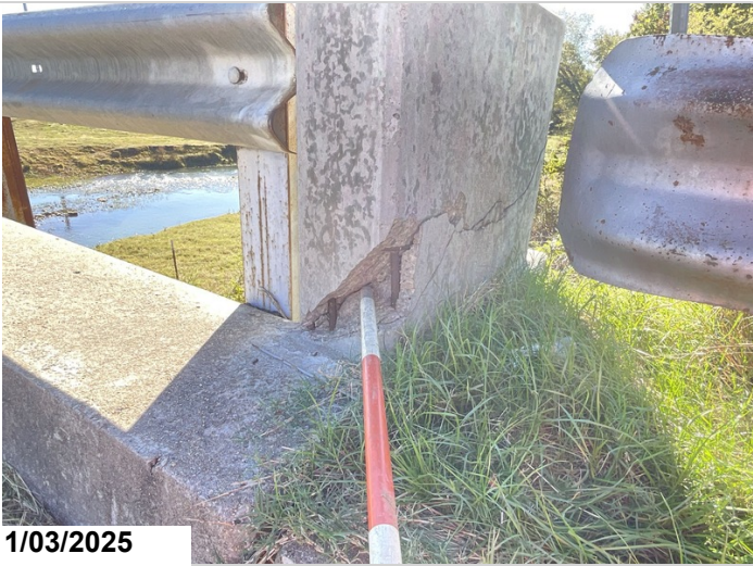
Abutment # 1, Right End Post: Fractured at the base with spalling that exposes reinforcing steel. Damage 1LF CS4.
