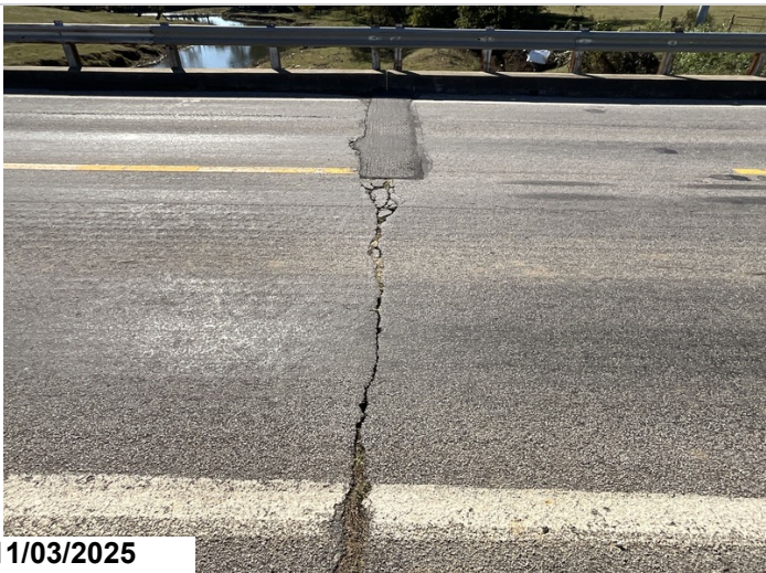
Bent # 2 Expansion Joint: Asphalt breaking apart.
