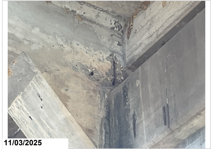
Span # 5, Bent # 6, Girder # 3: Shallow spalls with exposed reinforcing steel. Exposed steel 1LF CS3.
