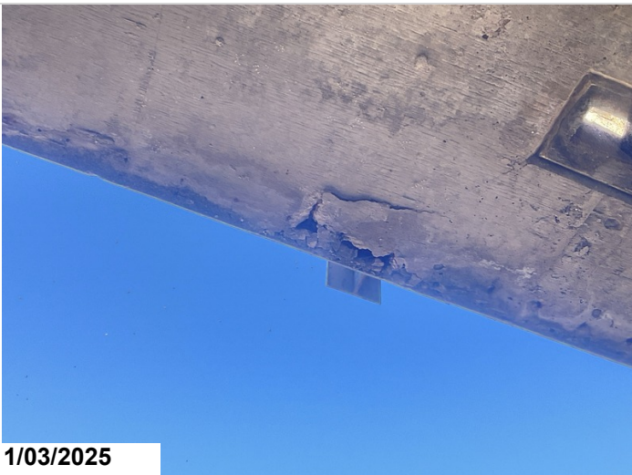
Span # 8, Left Deck Overhang: Spall/ delaminated area with exposed reinforcing steel. Exposed steel 1SF CS3.
