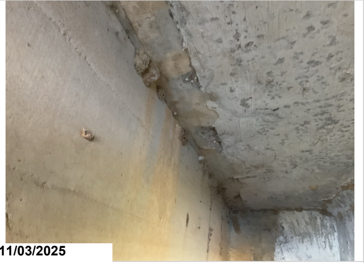
Span # 1, Bay # 1: Shallow spalling along Girder # 2 where the structure was widened. Spall/delam 10SF CS2.
