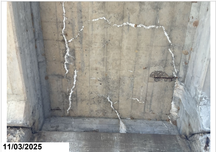
Span # 2, Bay # 2, At Bent # 2: Spalls with exposed reinforcing steel and cracking with efflorescence. Exposed steel 2LF CS3.
