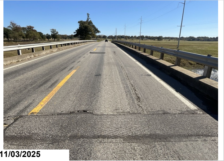
Right Lane: Asphalt patches over expansion joints.
