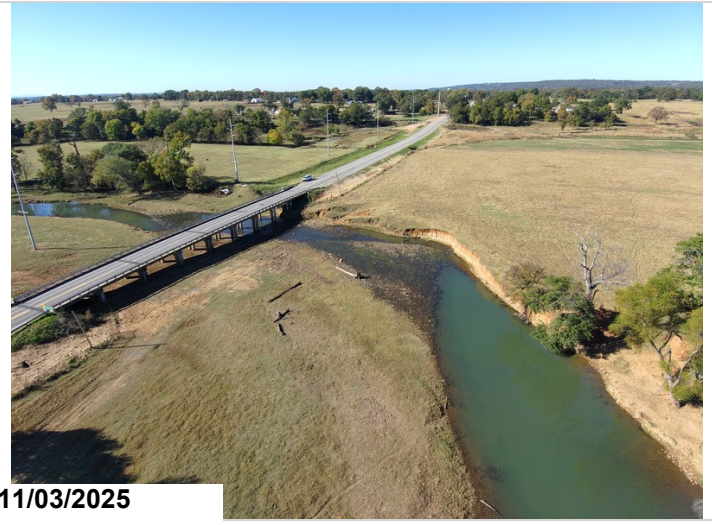
Embankment erosion upstream. Drone photo.
