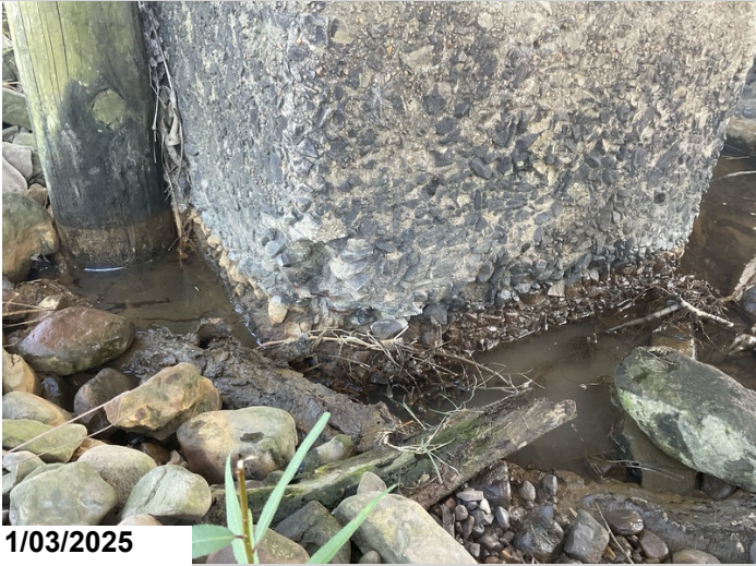
Bent # 5, Column # 1: Concrete deterioration with exposed steel. Exposed steel has complete section loss. Exposed steel 1EA CS3
