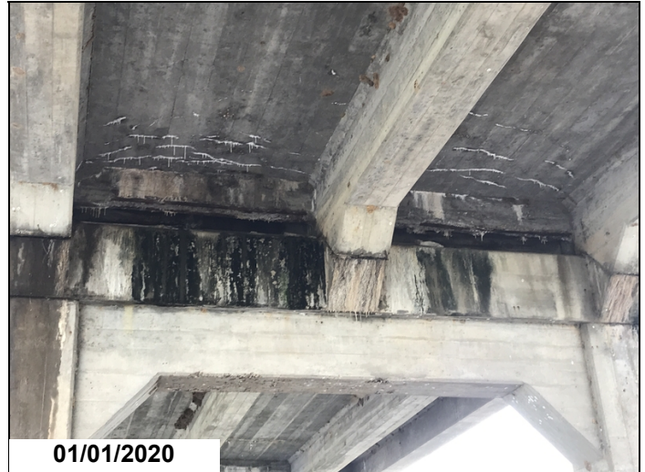
Bent # 4 spalling with exposed reinforcing steel in the expansion dam.
