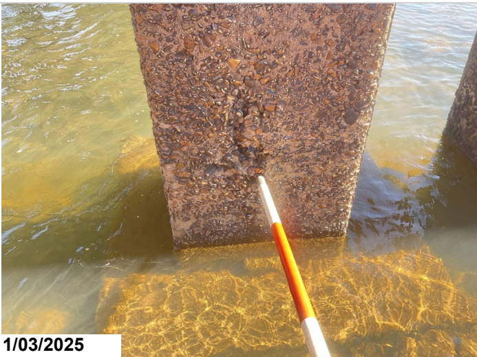
Bent # 3, Column # 3: Light abrasion with area of concrete deterioration. Spall/ delam 1EA CS3.
