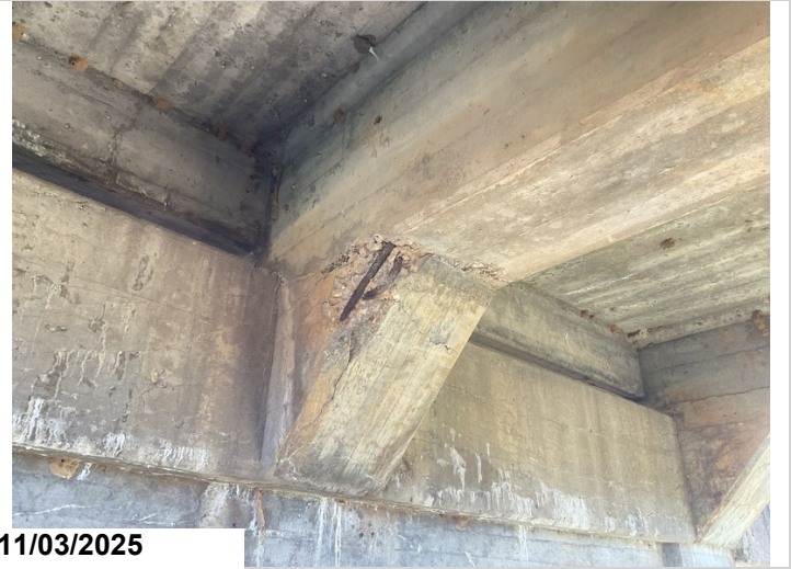
Span # 1, Girders # 3 and 4, At Bent # 2: Mapcracking in haunch, girder # 3 has spalls with exposed steel. Cracking 1LF CS3, Exposed steel 1LF CS3.
