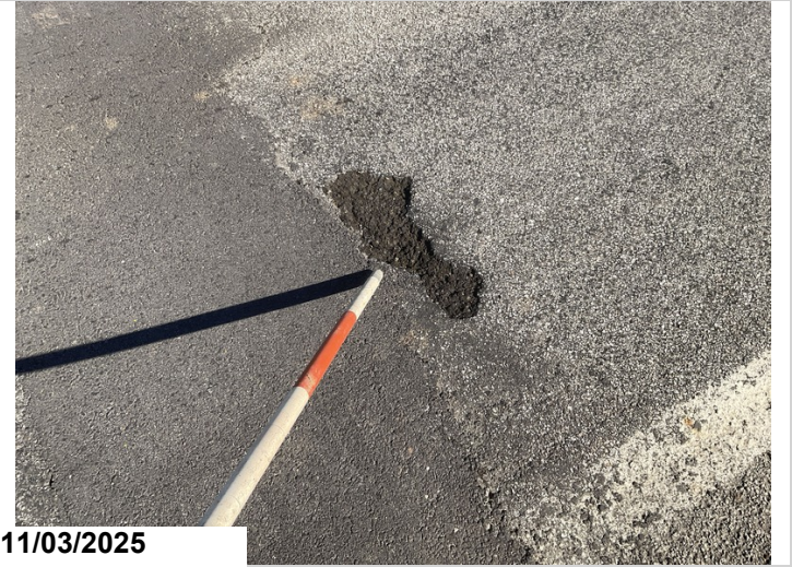
Span # 4, Right Lane, At Bent # 4: Pothole. Spall/ delam 2SF CS3.
