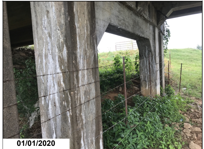
Bent # 2, columns # 2 & 3 have cracking with efflorescence.
