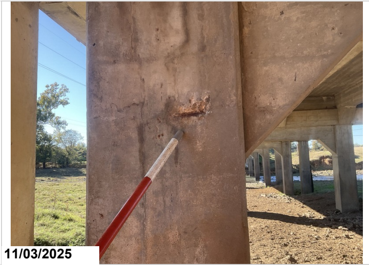
Bent # 8, Column # 3, Ahead Side: Spall with exposed reinforcing steel.
