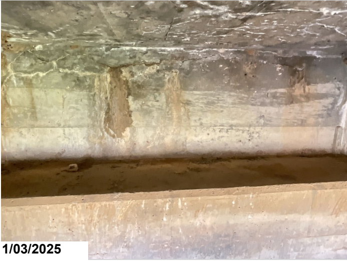
Abutment # 2 Back wall, Bay # 2: Moderate width horizontal cracking with efflorescence near deck juncture. Efflorescence 3LF CS2, Cracking 2LF CS2, 2LF CS3.
