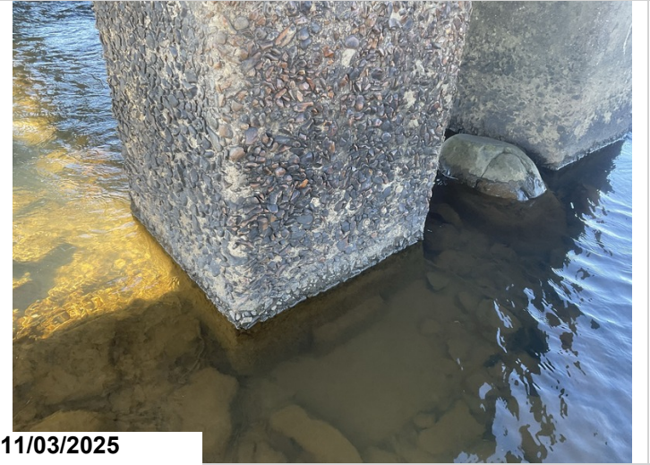
Bent # 4, Column # 2: Medium/ heavy abrasion. Abrasion 1EA CS3.
