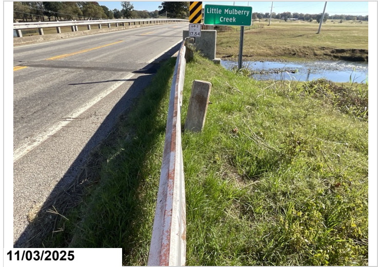
Abutment # 1 right approach railing has a failed bolted connection that attaches the railing to a post.
