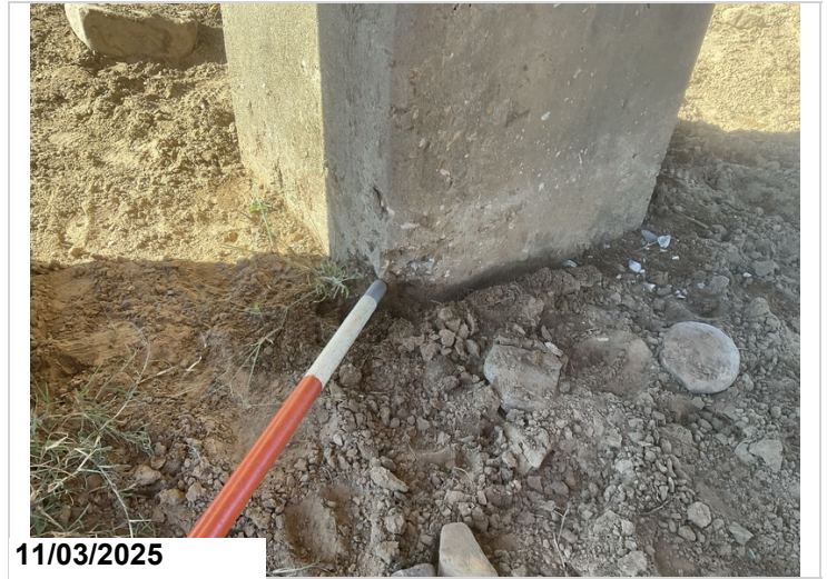
Bent # 8, Column # 3, Ahead Side: Spall at base with no exposed reinforcing steel.
