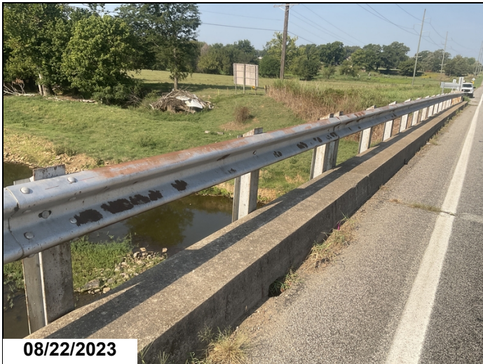
Bridge railing protective coating failing.
