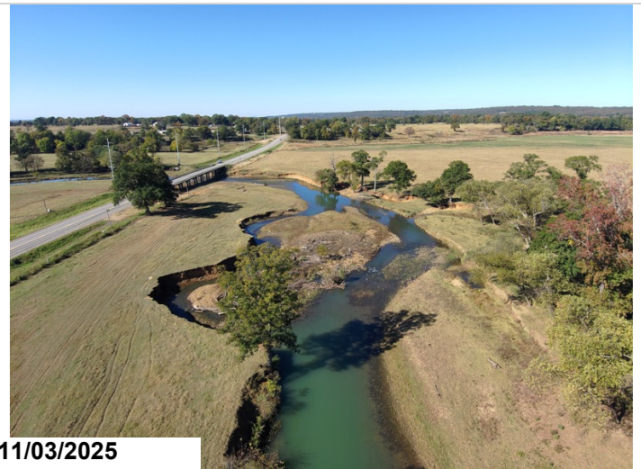
Embankment erosion upstream. Drone photo.
