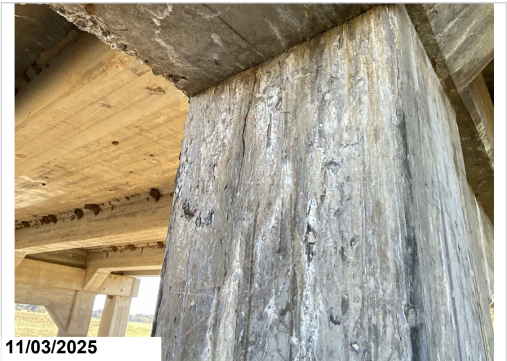
Bent # 2, Columns # 2 & 3: Map cracking and delaminated areas with efflorescence. Bent # 2, column # 2 has numerous vertical cracks with efflorescence with a 30" delaminated area in the exterior face near cap juncture. Cracking 2EA CS3.
