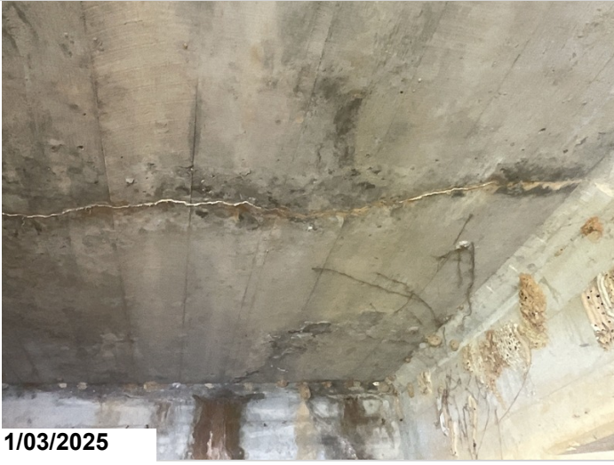
Span # 1 Undersurface, Bay # 1, 4' From Abutment # 1: Transverse crack with light efflorescence/ staining. 7SF CS3.
