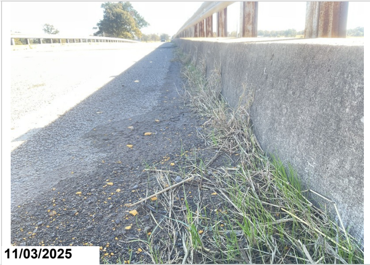
Shoulders have dirt and gravel accumulation with vegetation growing.
