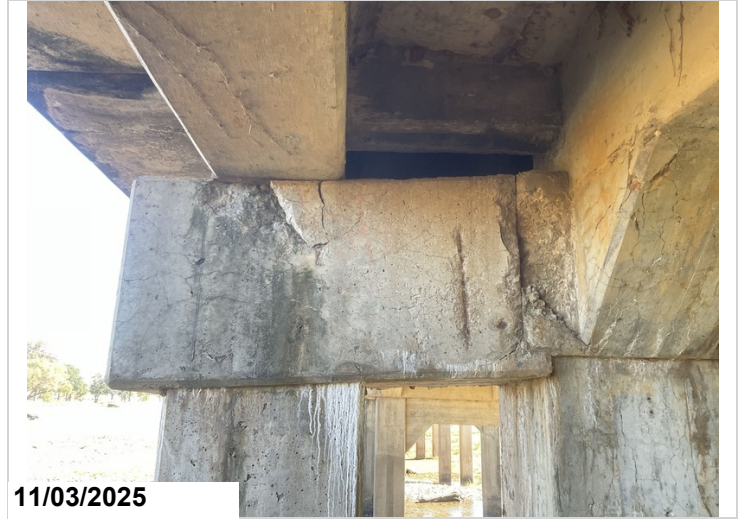
Bent # 2 Cap, Left Back Side: Spall/ delaminated areas and exposed steel. Spall/delam 1LF CS2, 2LF CS3, Exposed steel 1LF CS3.
