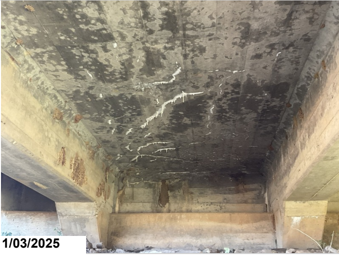
Span # 9 Undersurface, Bays # 2, Near Abutment # 2: Area of mapcracking with efflorescence. Cracking 48SF CS3.
