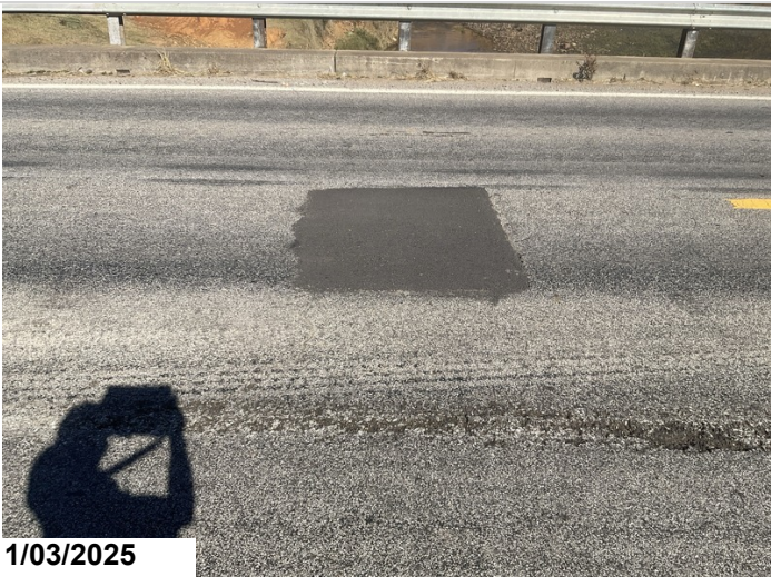
Span # 3, Over Bent # 2: Asphalt patch. Spall/ delam 16SF CS2.
