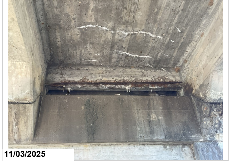
Span # 8, Over Bent # 8, Bay # 2: Spalling with exposed reinforcing steel. Exposed steel 7SF CS3.
