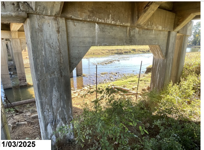
Bent # 2, Columns # 2 & 3: Map cracking and delaminated areas with efflorescence. Bent # 2, column # 2 has numerous vertical cracks with efflorescence with a 30" delaminated area in the exterior face near cap juncture. Cracking 2EA CS3.
