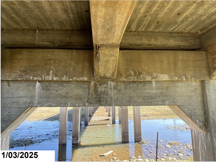
Bent # 2 Cap, Back Side: Mapcracking with efflorescence cracking 11LF CS3.
