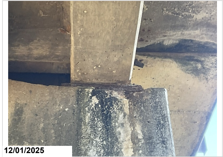
Bents # 2 Ahead Side, Bearing # 1: Bearing has corrosion with flaking rust/ section loss. Cap has shallow spalling with minor loss of bearing area to the masonry plate of bearing. Corrosion 1EA CS3.
