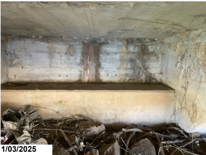
Abutment # 1 Backwall, Bay # 2: Vertical and diagonal cracking with efflorescence and rust staining. Efflorescence/staining 3LF CS3.
