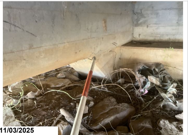
Span # 1, Girder # 3, Abutment # 1: Delaminated area. Spall/delam 1LF CS2.
