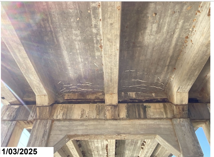
Span # 4, Bays # 2 and 3, At Bent # 4: Mapcracking with efflorescence. Cracking 48SF CS3.
