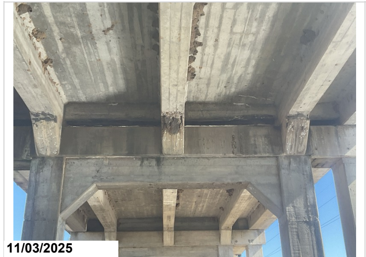
Span # 3, At Bent # 4: Spalling in ends of girders at haunch interface. Exposed steel 4LF CS3.
