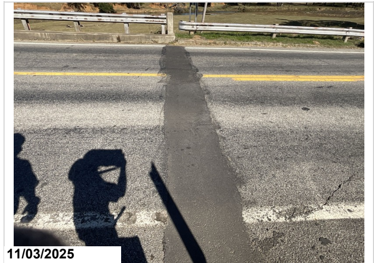
Abutment # 2, Expansion Joint: Asphalt patch.
