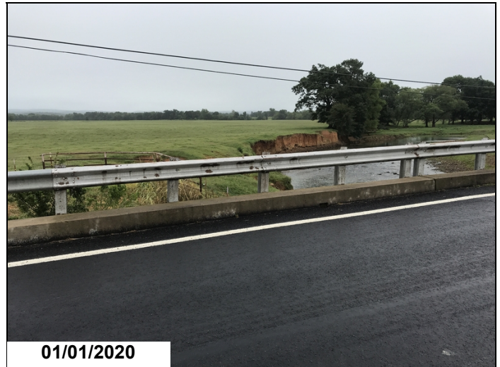
Bridge railing protective coating failing.
