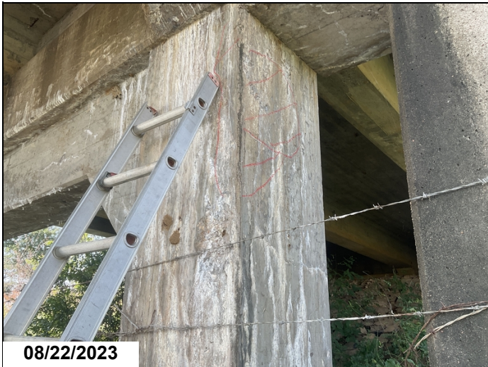
Bent # 2, column # 2 has numerous vertical cracks with efflorescence and a 30" delaminated area in the exterior face near cap juncture.
